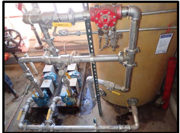
Photo 28 Hangar 133 AFFF pump and activation system.
