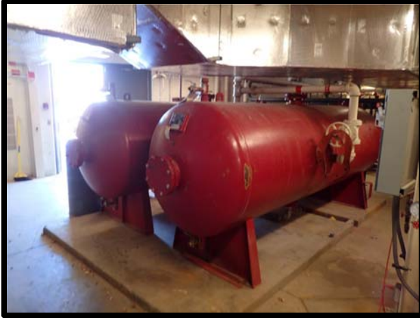
Photo 73 Hangar 210 AFFF storage tanks.
