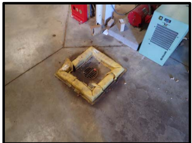
Photo 72 Drain protection in place at Hangar 210.
