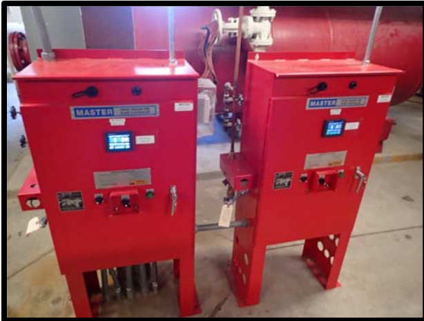
Photo 75 Hangar 210 diesel engine pump controllers.
