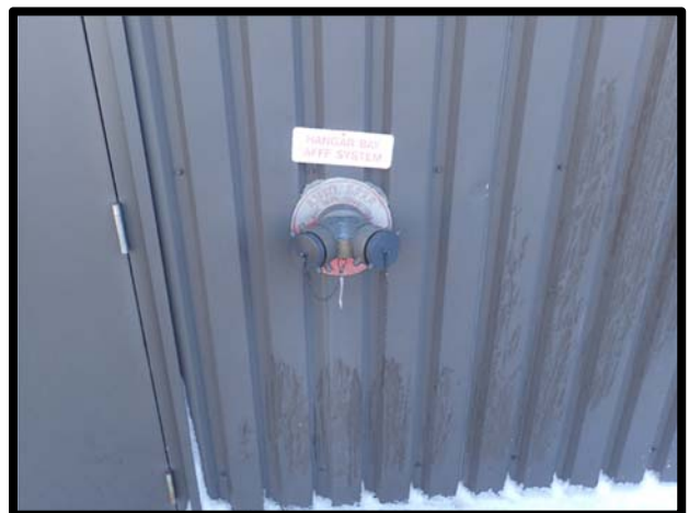
Photo 42 Fire department connection to AFFF system at Hangar 121.
