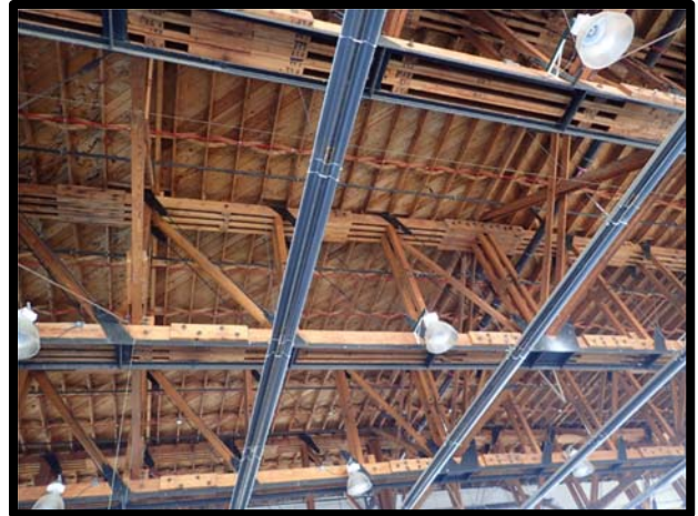
Photo 32 Ceiling joists and AFFF suppression system at Building 131.
