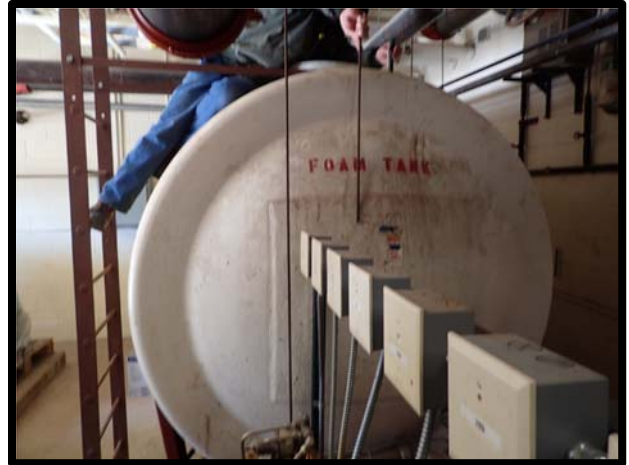
Photo 56 Showing the level of AFFF concentrate at Hangar 214.
