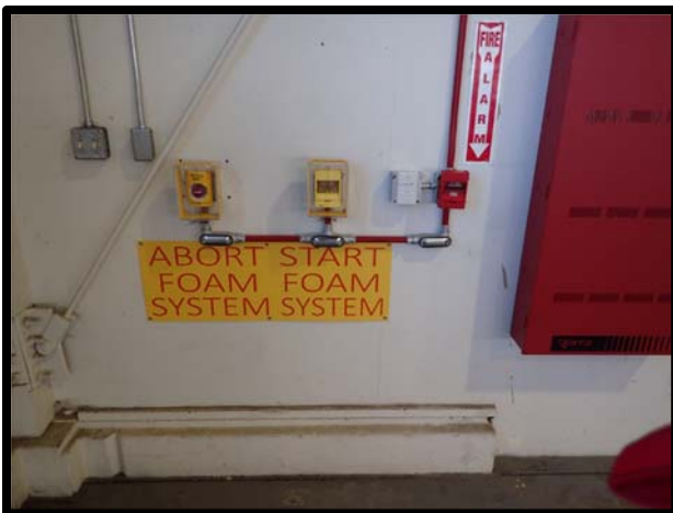
Photo 47 Hangar 121 foam controls.
