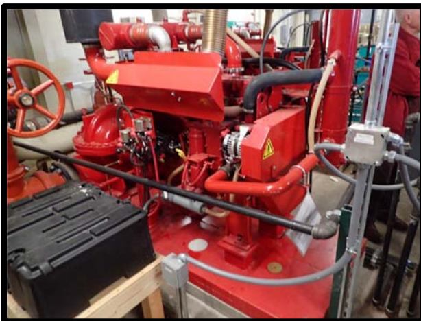
Photo 76 Second view of Hangar 210 diesel pumps.
