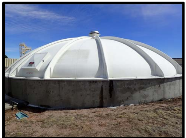
Photo 96 Current FTA used water holding tank.
