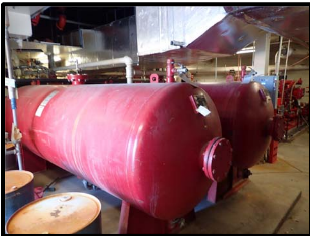
Photo 69 Hangar 210 AFFF storage tanks.
