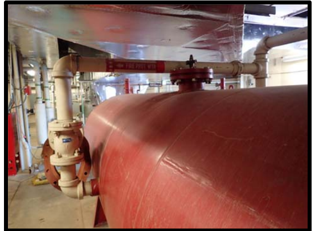
Photo 76 Hangar 210 fire suppression water supply to AFFF tanks.
