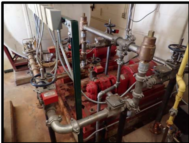
Photo 59 Foam pumping system at Hangar 214.
