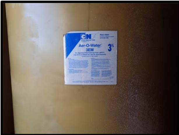
Photo 27 Hangar 133, 3 percent AFFF label on 800-gallon tank.
