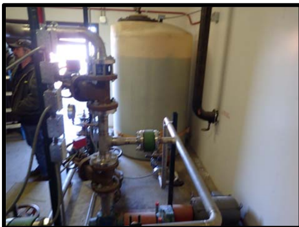
Photo 41 Hangar 121 AFFF activation system.
