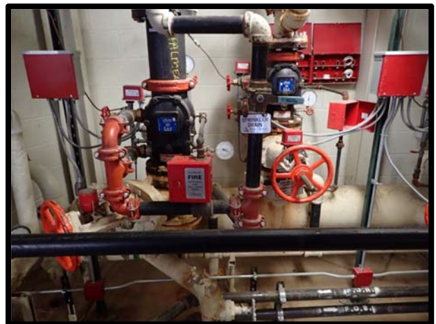
Photo 77 AFFF dispensing manifold in Hangar 210 mechanical room.
