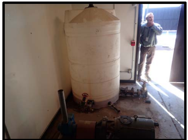
Photo 54 Decommissioned foam tank at Hangar 119.
