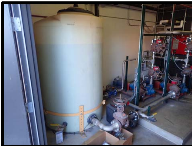
Photo 39 Hangar 121 AFFF storage tank, 600-gallon capacity.
