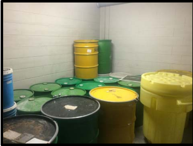
Photo 12 AFFF Storage at Fire Station #1, 600 gallons.
