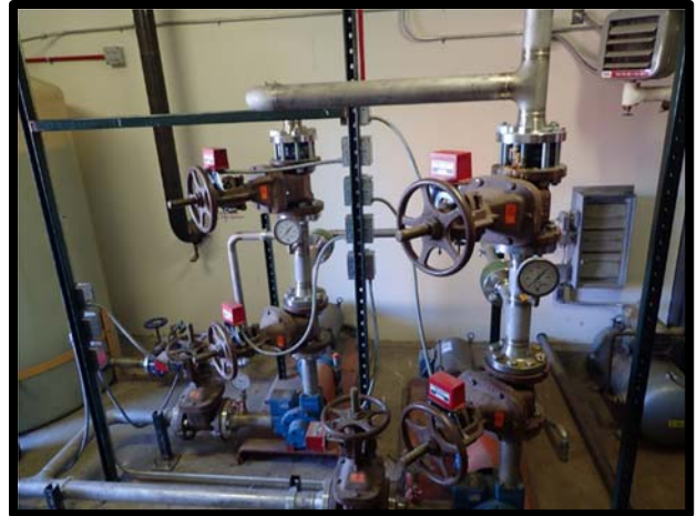
Photo 38 Hangar 121 AFFF activation system.
