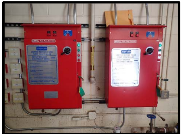
Photo 58 AFFF pump control system for Hangar 214.
