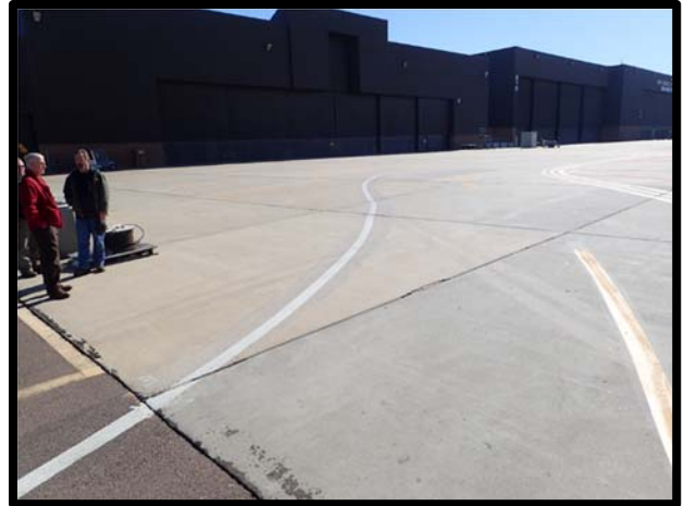
Photo 68 Southeast looking photo of Hangar 214. Note the good repair of the concrete.
