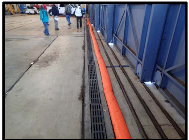
Photo 48 Deflated containment booms from AFFF system testing at Hangar 121.
