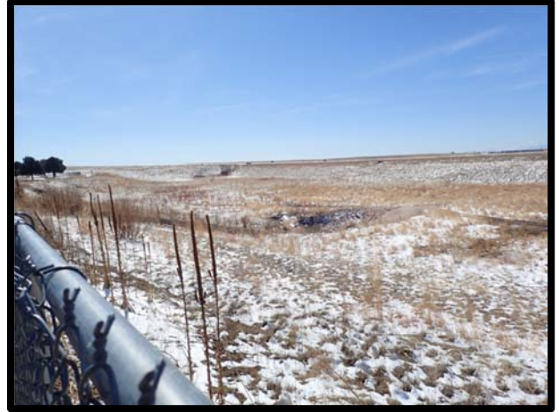
Photo 86 Unlined detention pond next to Pond #3. Notice the overflow scarring.
