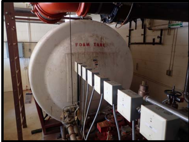
Photo 55 AFFF storage tank at Hangar 214 (2,000-gallon).
