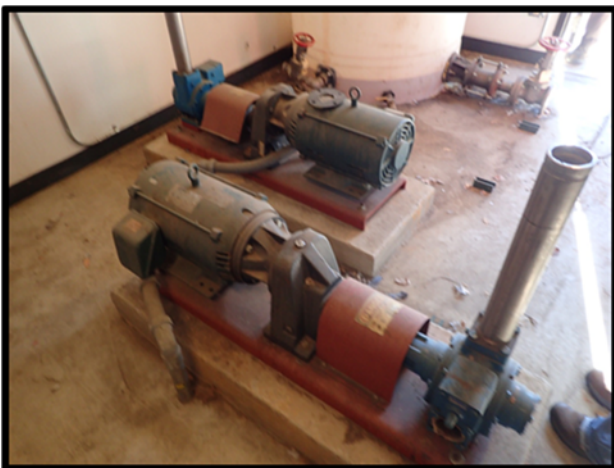
Photo 53 Decommissioned foam system at Hangar 119.
