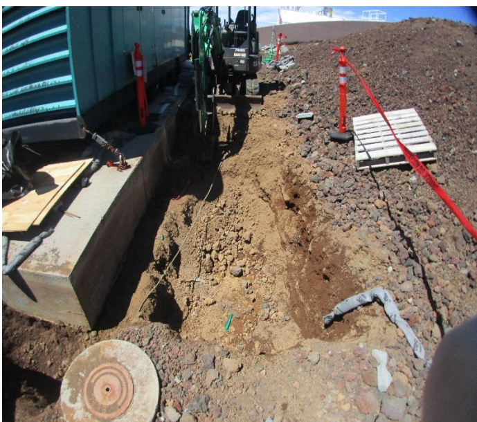
Photo 7: Site inspection; excavating 2 feet depth from northeast corner of generator pad. 3/10/23
