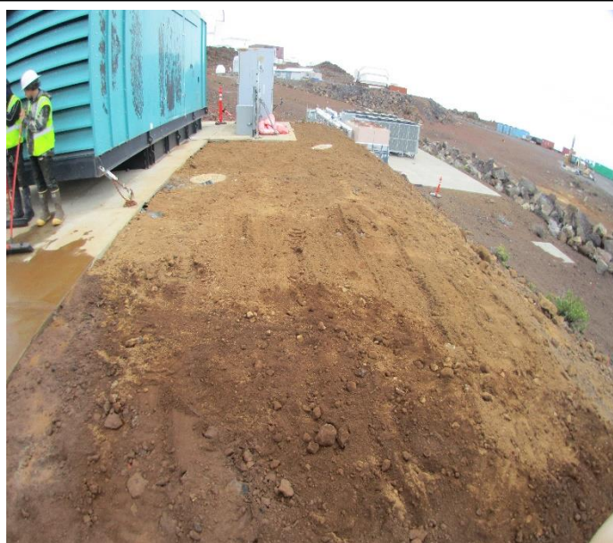
Photo 16: Excavation backfilled. 3/22/23
