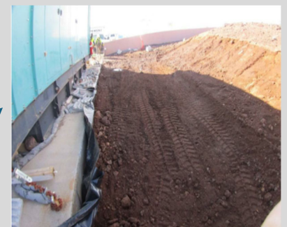
Same area after Phase 1 excavations
