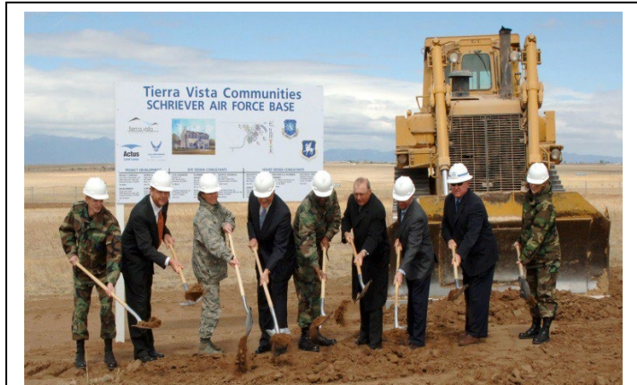
Col Theresa Djuric (third from left), 50 SW commander, and others, including representatives of Tierra Vista Communities, break ground on base housing, May 16, 2008 (USAF Photo)
